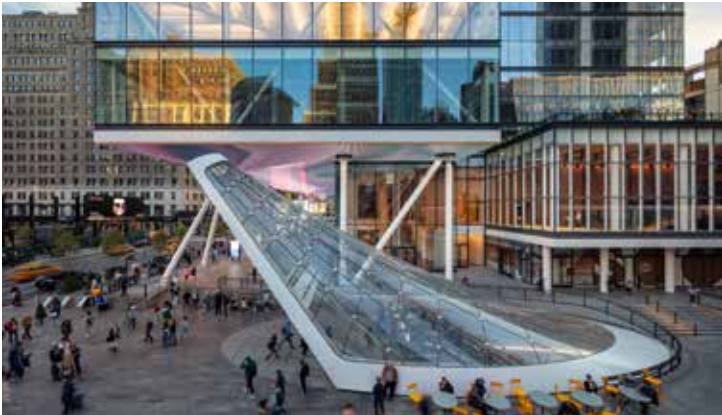
Metals in Construction & 2025 IDEAS² PENN 2
